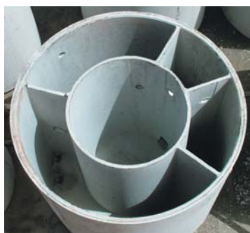
Completed Tank Ready for Fitout and Lid
