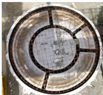
Inverted Mould with Reinforcing Ready for Concrete
